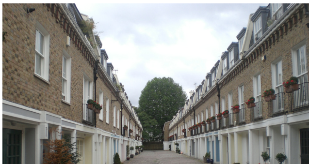
Figure 4.33: Consistent roofscape with regular rhythm of dormer windows
