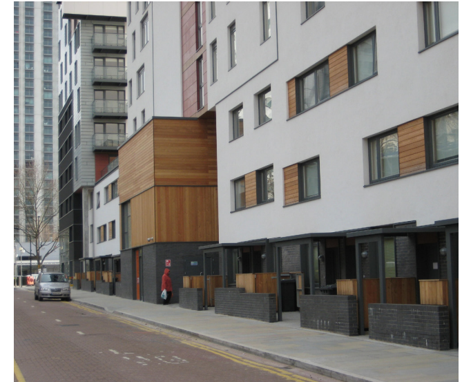
Figure 4.34: A development at Mastmaker Road with individual front doors for every ground floor flat.
