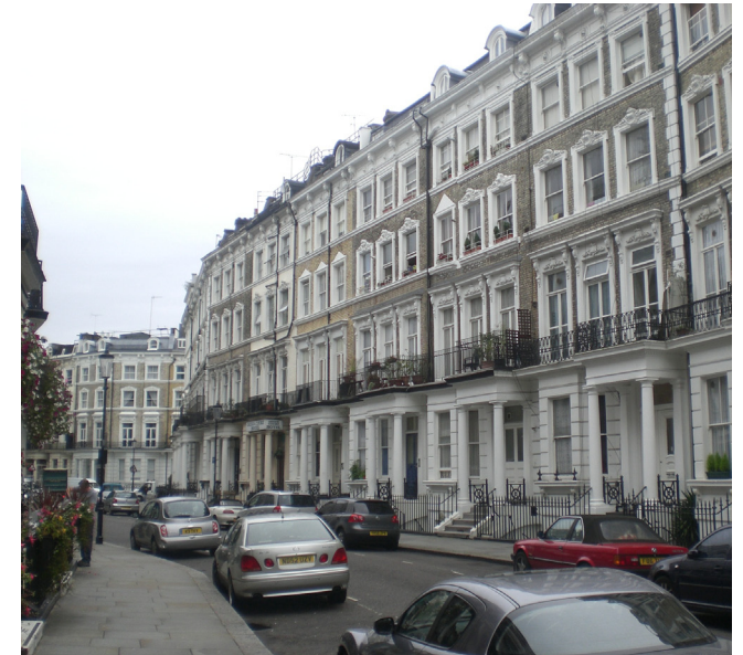
Figure 5.1: Photograph of terraced housing
