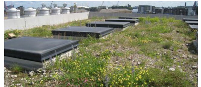
Figure 12.4: Photograph of a green roof
