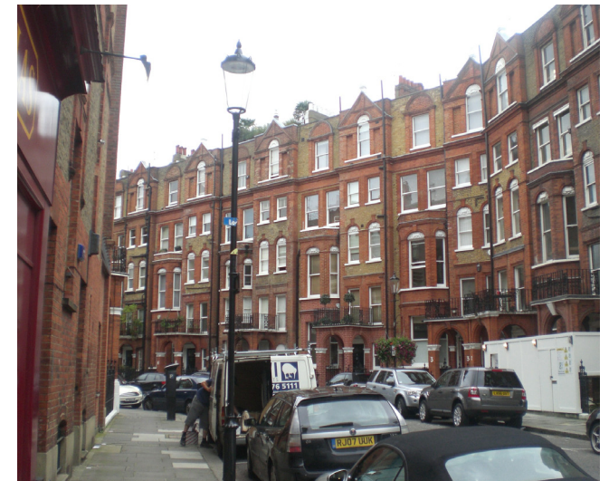
Figure 5.2: Photograph of mansion blocks
