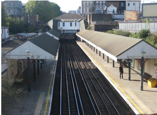
Figure 4.8: The railway line at the West Kensington platforms
