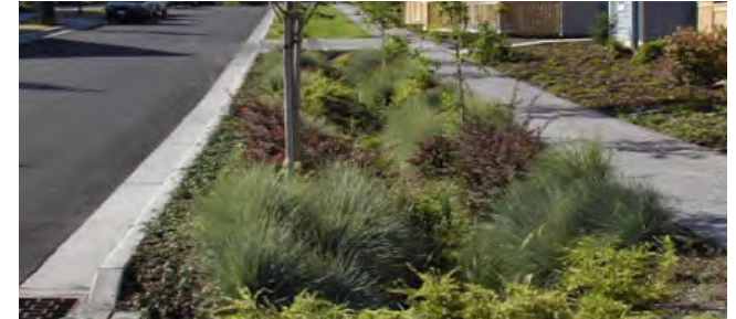
Figure 12.2: Photograph of landscaped drainage channels
