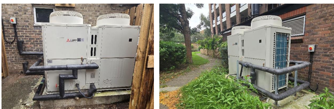
Heat pumps in place in communally-heated blocks
