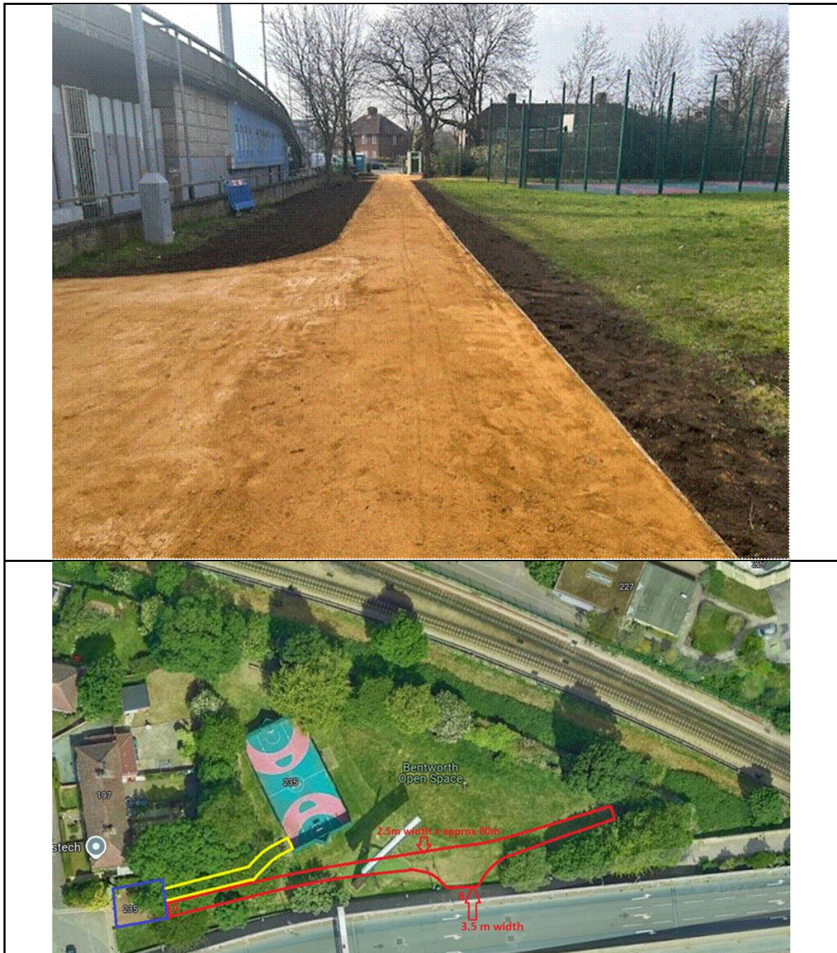
Figure .44: Creation of New Self Binding Aggregate Pathway at Bentworth Open Space.
