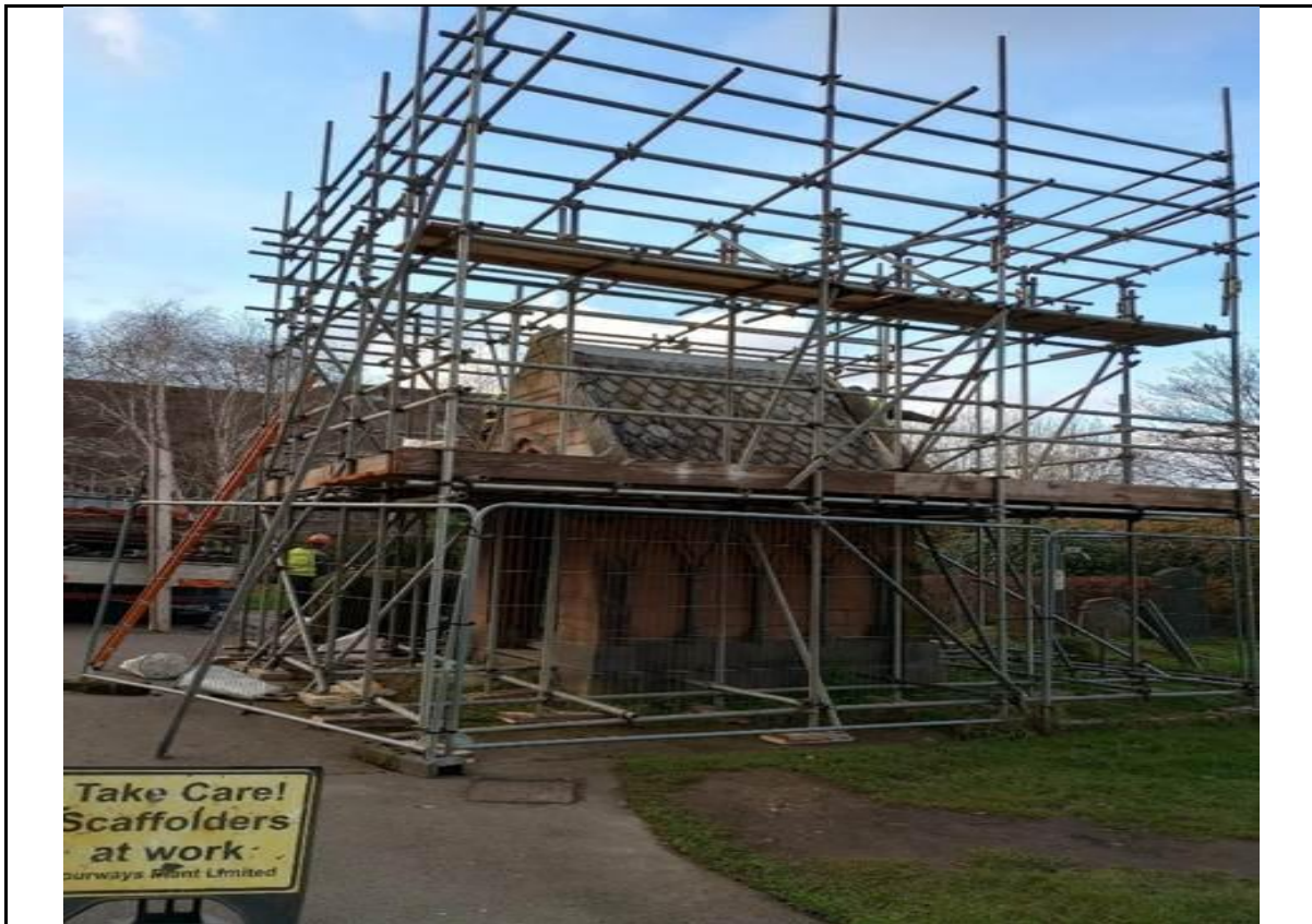
Figure 42: Scaffolding going up around the mausoleum.
