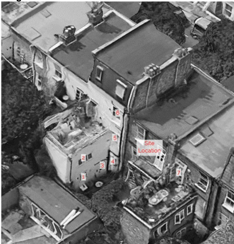
Image 1: Tested Windows at No.13 Eustace Road
