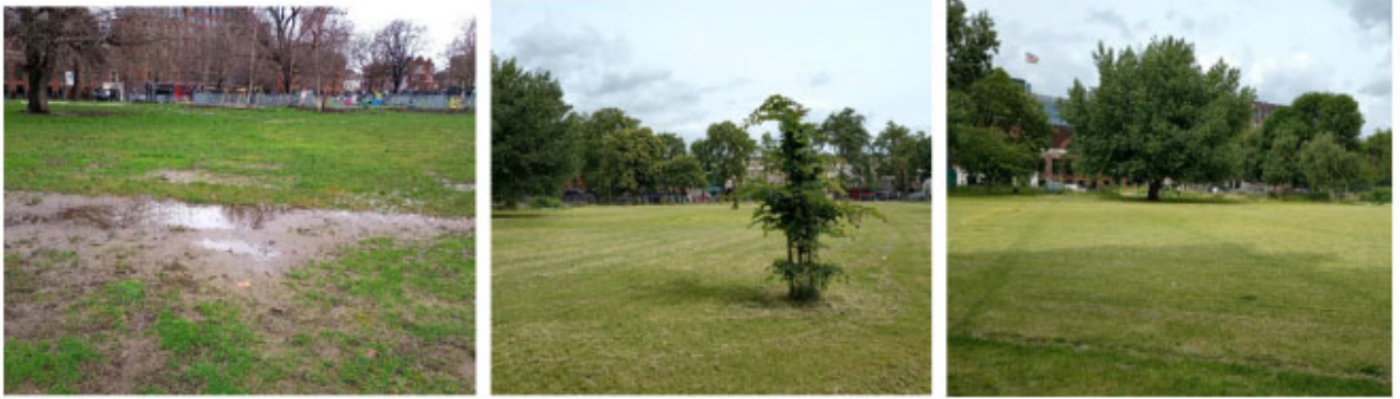
Figure 24: Shepherds Bush Green - Drainage works. Installed new land drains to the western field, which has been affected by surface water flooding during the winter months. The new system included underground drains, levelling the ground surface and grass seeding.
