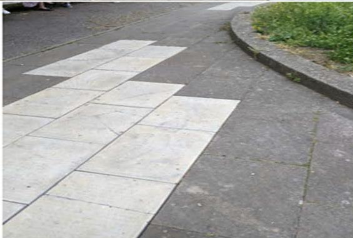
Figure 26: Paving and bins improvements at St. Paul's
