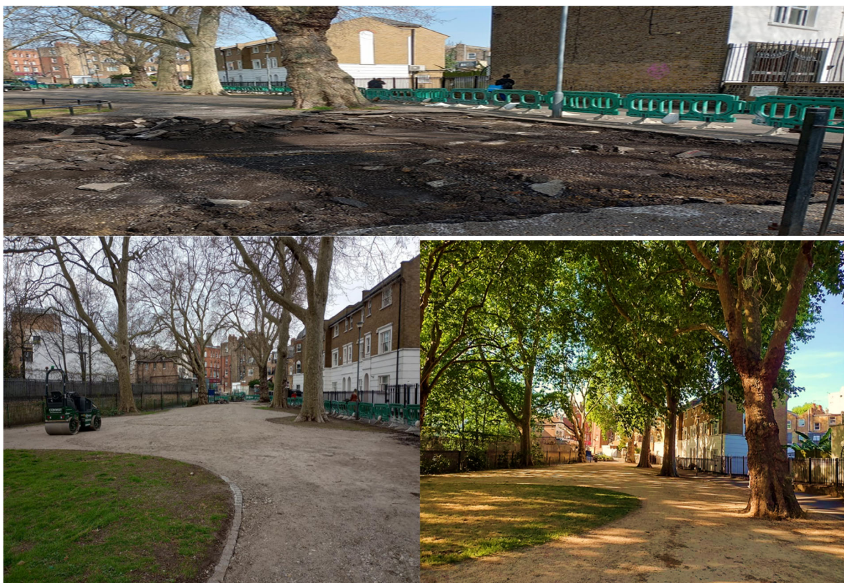
Figure 16: Footpath resurfacing of north area – ‘de-pave’ of macadam surface and reinstatement with self-binding aggregate at Eel Brook Common
