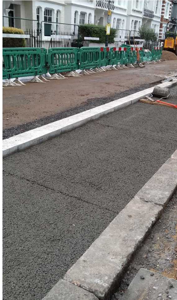
Figure 3: Just laid pervious concrete – Eddiscombe Road
