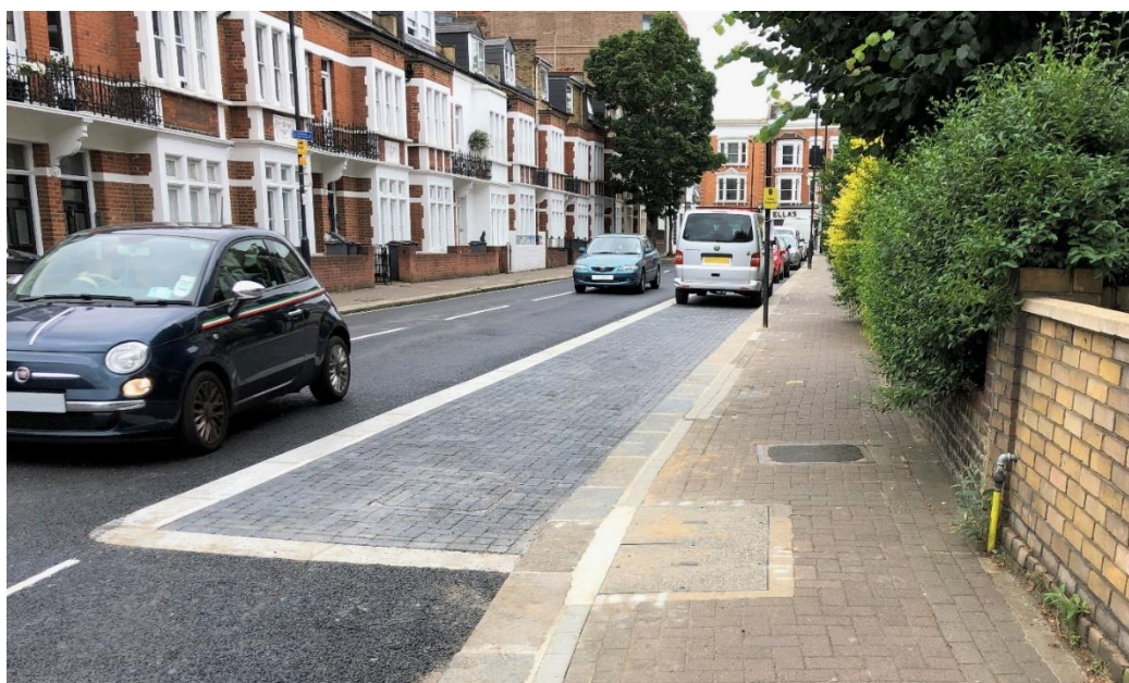
Figure 5: Finished scheme – Munster Road
