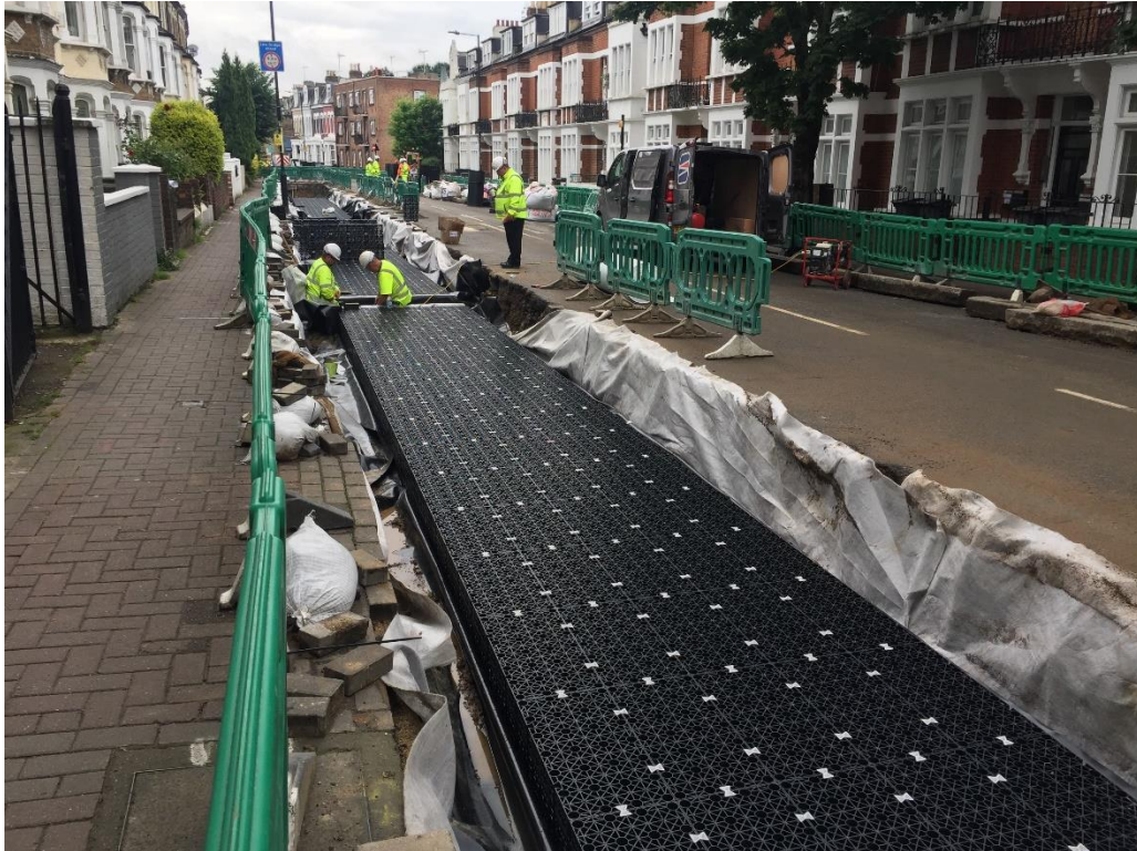
Figure 2: Installation of geocellular units on site – Munster Road
