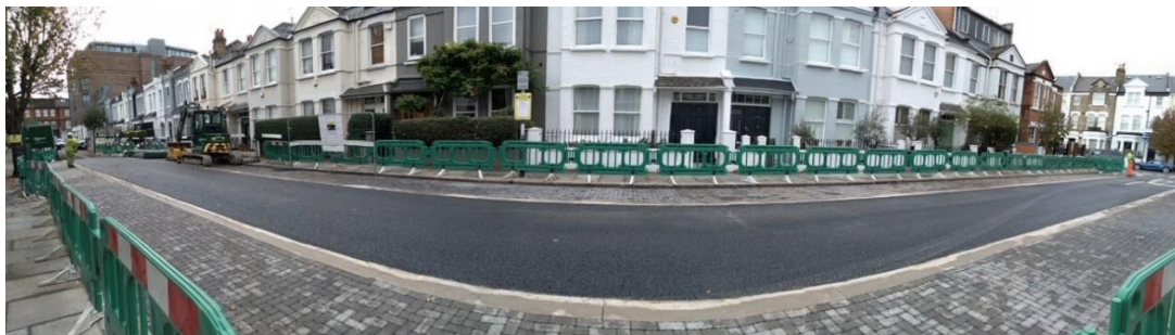
Figure 4: Finished scheme – Eddiscombe Road
