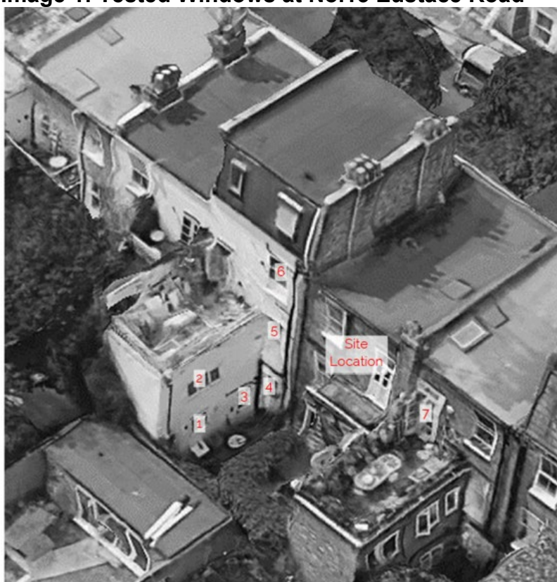
Image 1: Tested Windows at No.13 Eustace Road
