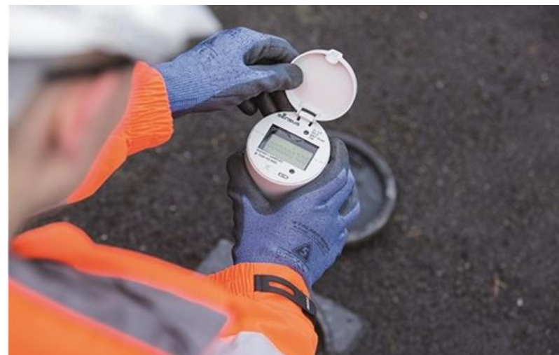
Image 4: Fitting a water meter
