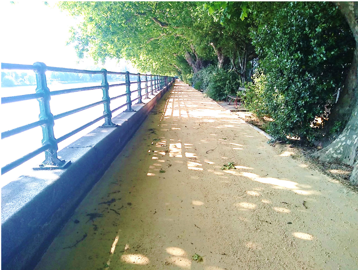
Figure 11: Bishops Park – Footpath resurfacing along the riverside. Previous macadam surface was de-paved and replaced with a self-binding aggregate material.
